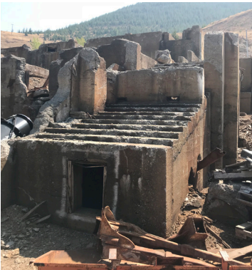
View of the former zinc plant area.
