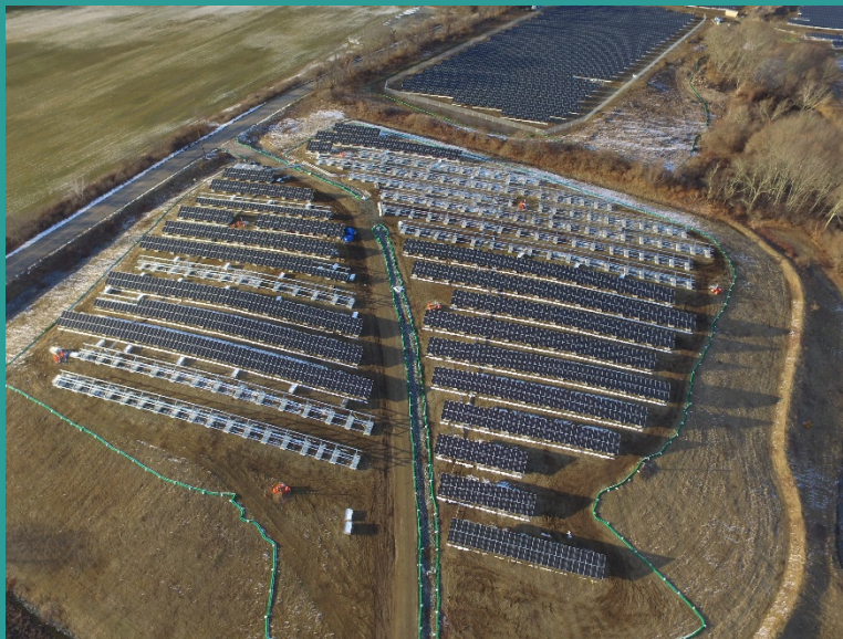
Aerial view of the West Kingston Town Dump/URI Disposal Area site. Image used with permission of Kearsarge Energy.
