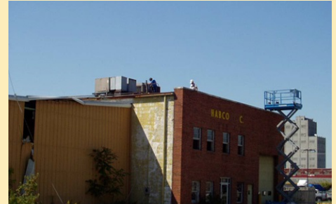
The former Habco building demolished during the first removal action.
