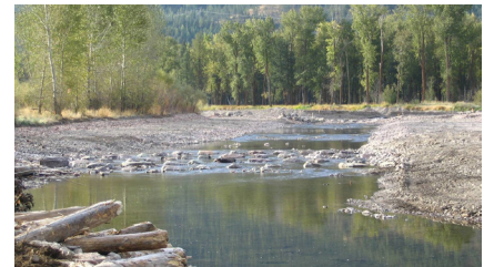
View of the restoration channel and shaping grade control dam.
