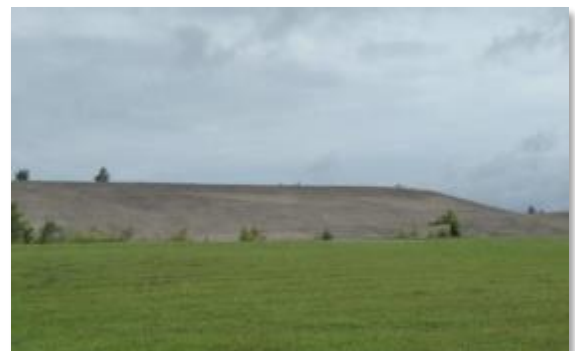
Figure 3. Mine tailings piles, such as the one above, are located throughout the response area.
