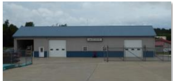
Figure 10. A warehouse on the Waterworks Specialties company property.
