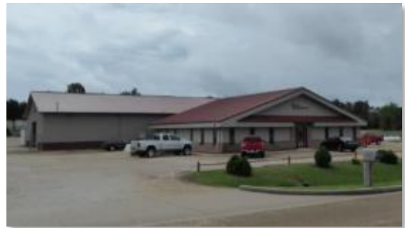
Figure 8. GWS Contractors, Inc. operates out of this facility.
