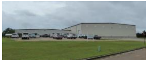
Figure 9. Trelleborg opened its new facility in Bonne Terre in 2017.
