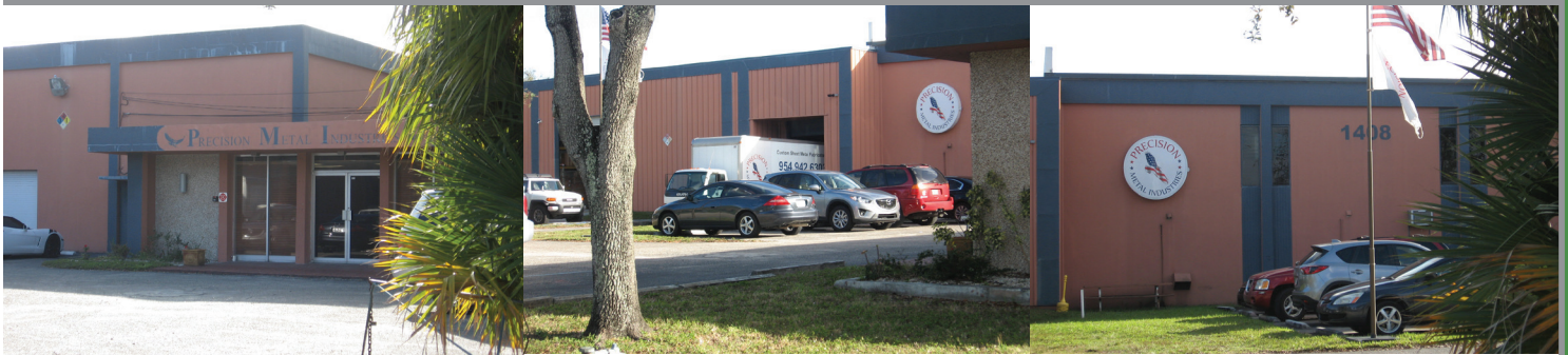
Images from left to right: Views of the Precision Metals Industries building and parking area.
