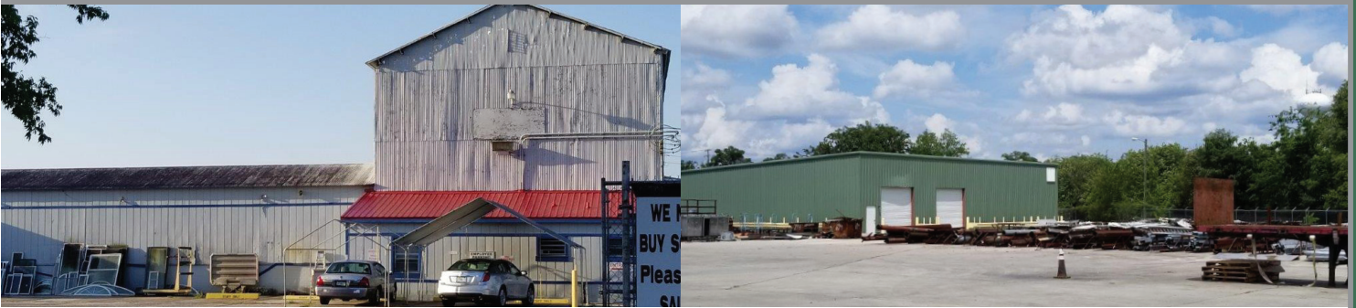
Views of the scrap metal recycling facility.
