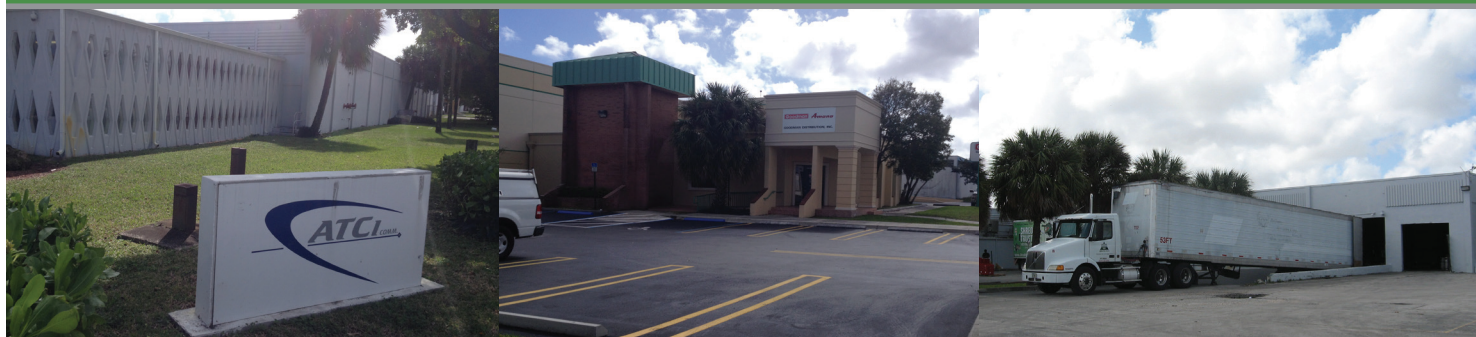
Images from left to right: The ATCI International Global Security building, Goodman Amana facilities and a loading dock at the site.
