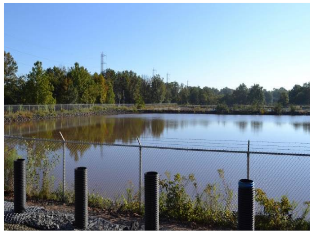
Figure 3. Waste disposal impoundments at the site will be remediated using methods that will allow for security in the face of storm or flooding impacts.
