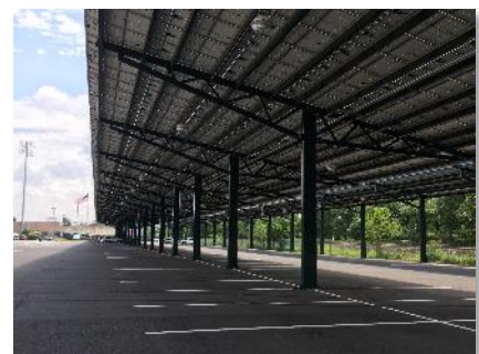
Figures 7, 8 and 9. The TD Bank Ballpark is next to New Jersey Transit's Bridgewater Station. When not in use for stadium games and events, the parking lots are used for commuter parking. Two parking lots at the stadium have elevated solar panels that generate clean, renewable energy for the stadium and provide shaded parking spaces.
