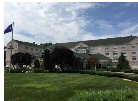
Figure 12. Front view of the Hilton Garden Inn located on-site.
