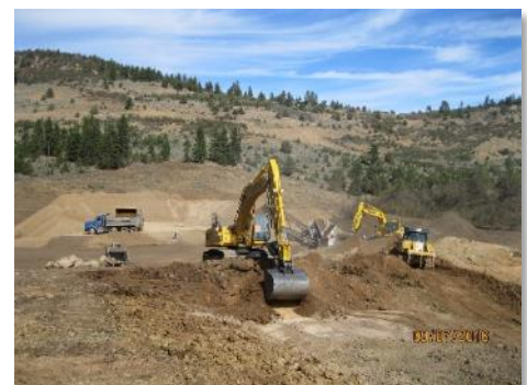
Figure 8. Collecting clean fill from the nearby borrow area.
