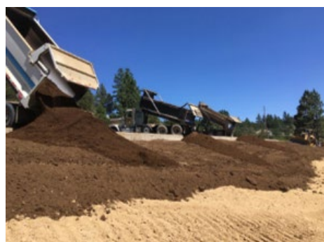
Figure 5. Filling to grade with clean soil.
