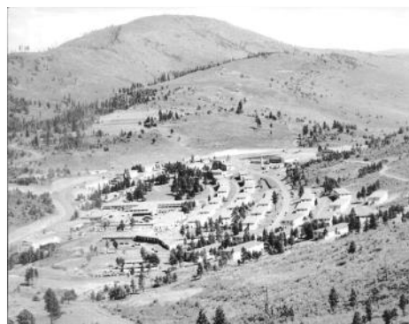
Figure 3. The former Marine barracks, prior to demolition.
