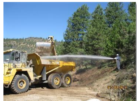
Figure 14. Remediation worker on site.
