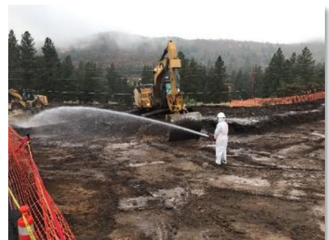
Figure 10. Worker in personal protective gear.
