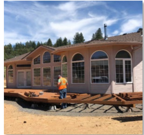
Figure 7. Installing new home decks at the site.
