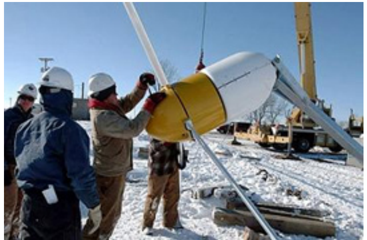
Figure 13. Installation of the wind turbine system at the Former Nebraska Ordnance Plant site (Nebraska).
