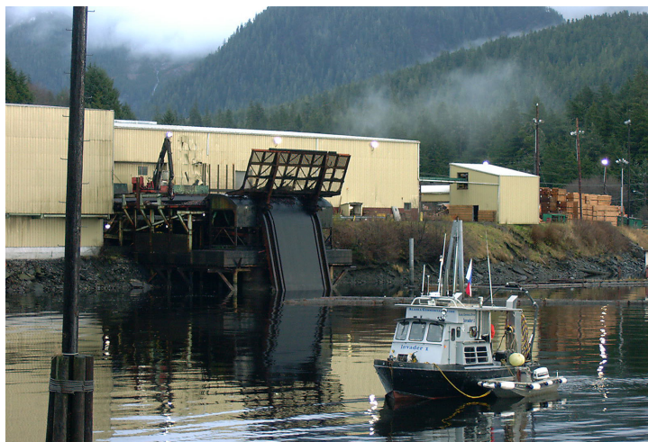
Figure 2. Log lift used to remove bundled logs from the water at the Ketchikan Pulp Company site (Alaska).
