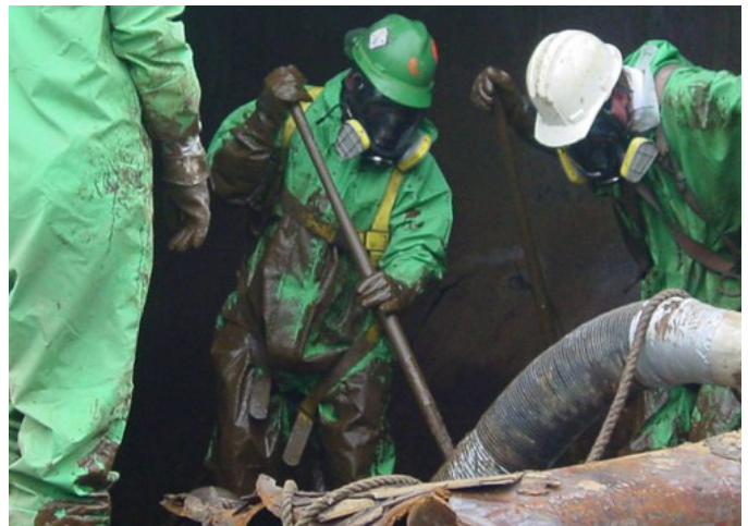
Decontamination of a tank.
