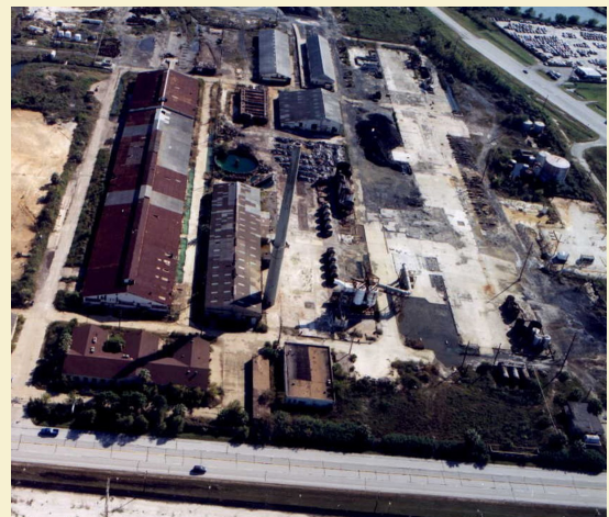
The Tex Tin Corp. Superfund site before cleanup.
