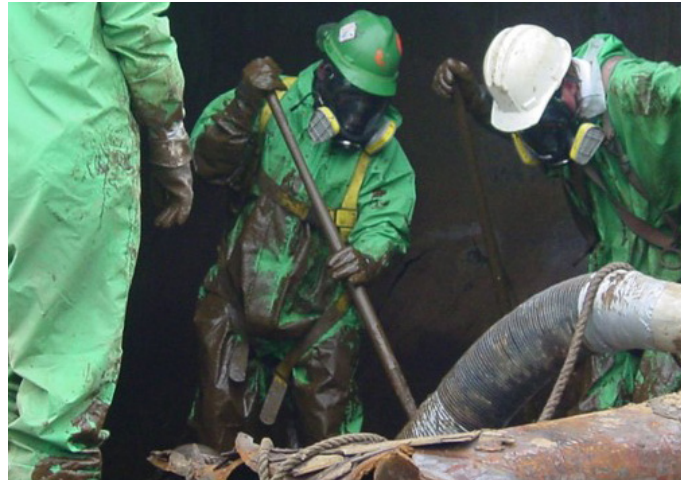
Decontamination of a tank.
