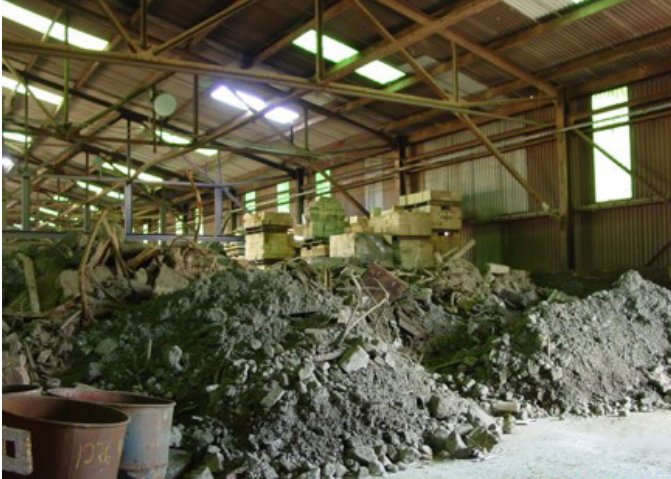
Original site conditions in the ore storage building.
