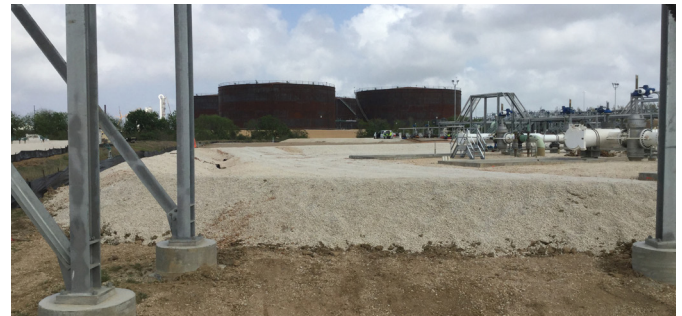
Construction of tanks and equipment at the Texas City Terminal.
