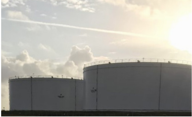
The Texas City Terminal's oil storage tanks were placed on top of capped areas.
