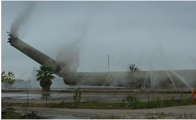
Demolition of the original smelter stack at the site.
