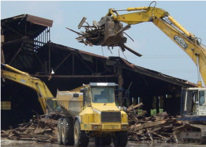
Demolition of the ore storage building.
