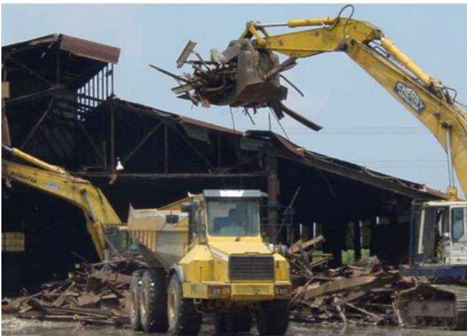
Demolition of the ore storage building.
