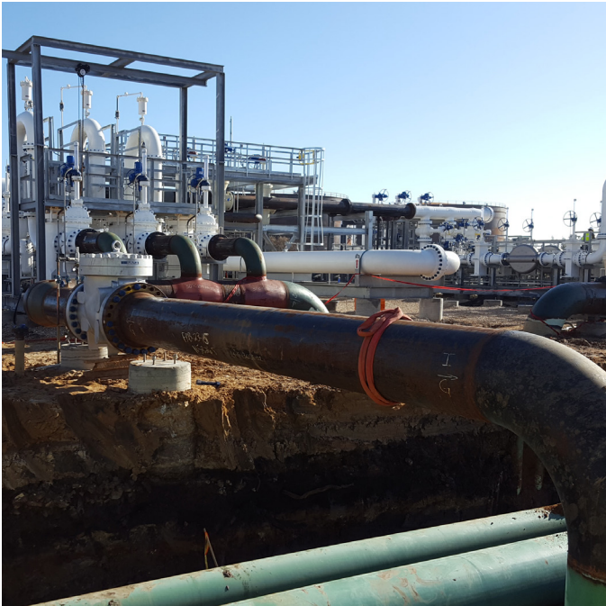
Genesis' construction of the Texas City Terminal.
