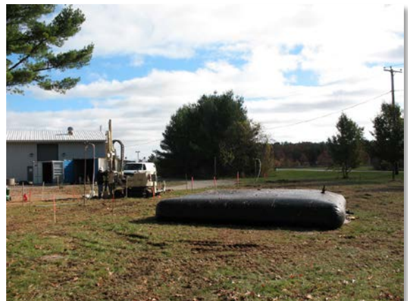
Figure 3. Bioremediation injection at the site.
