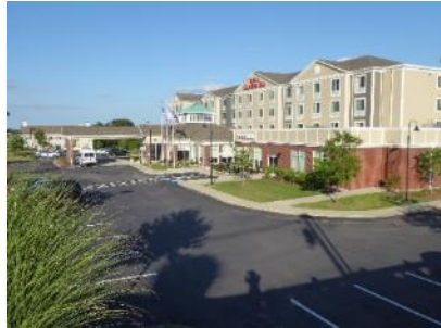
Figure 13. The Hilton Garden Inn was built on site in early 2016.
