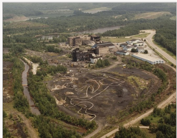
Aerial view of the J&L Steel Site (2016) showing State Highway 3, the upper facility and petroleum spill area.
