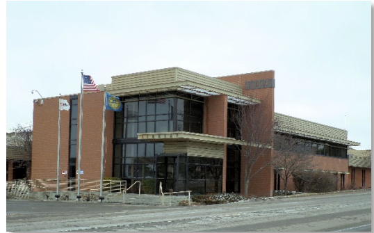
Figure 5. Lindsay Manufacturing's offices on site.
