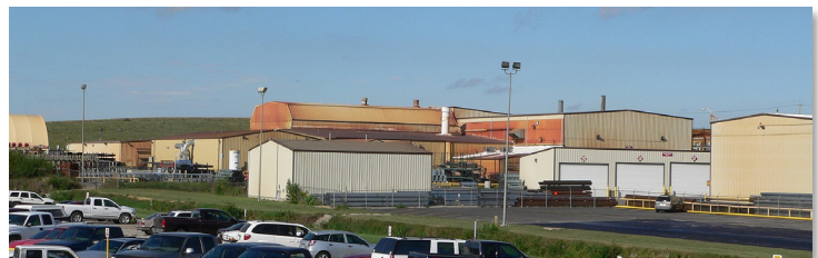
Figure 4. Lindsay Manufacturing Co. facility as seen from the southwest.
