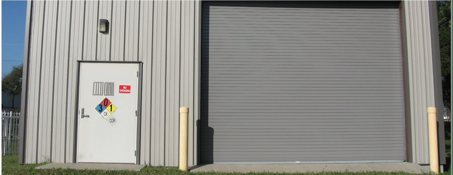
Exterior of the groundwater treatment plant building.
