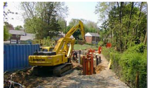
Figure 4. Cleanup activities at the Havertown PCP site.
