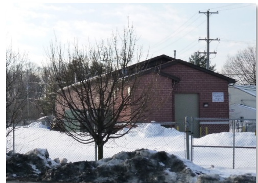
Figure 5. Groundwater treatment facility on the north end of the site.
