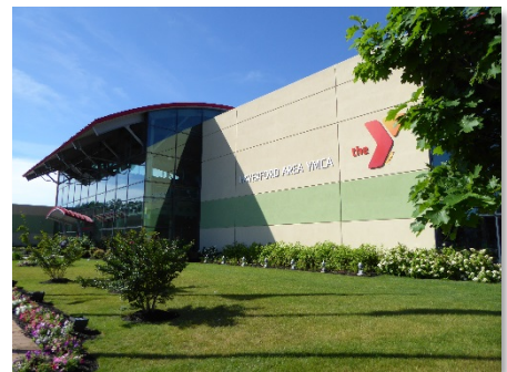
Figure 1. New Havertown Area YMCA facility.
