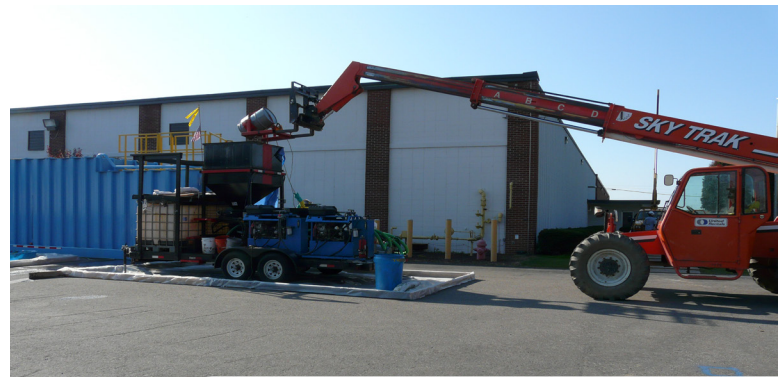
Chemical oxidation injections into site groundwater are part of site cleanup efforts.
