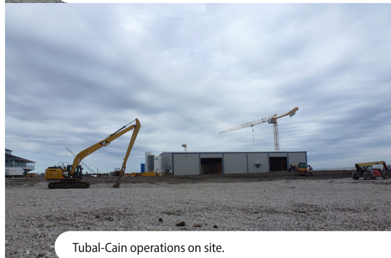
Tubal-Cain headquarters on site.
