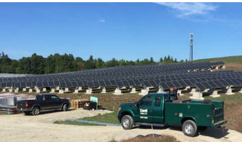
A view of completed installation of panels.
