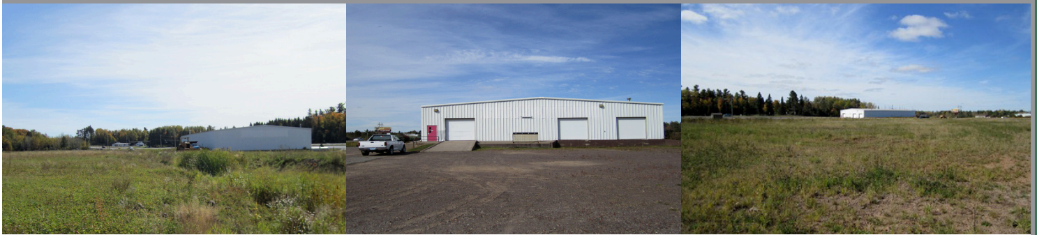
Images from left to right: Views of a warehouse and land available for development on site.
