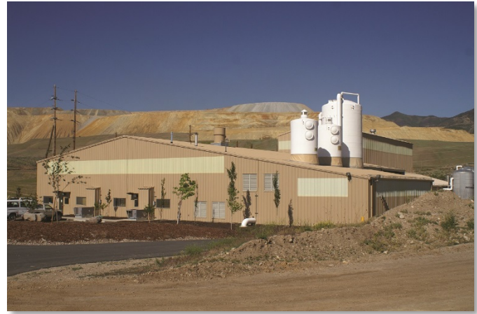
Figure 5. One of the site's two groundwater treatment plants. (Image source: Rio Tinto)
