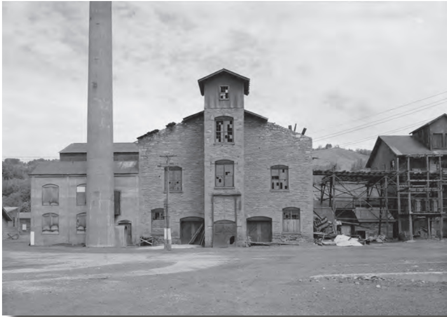
View of the main smelter facility prior to cleanup.
