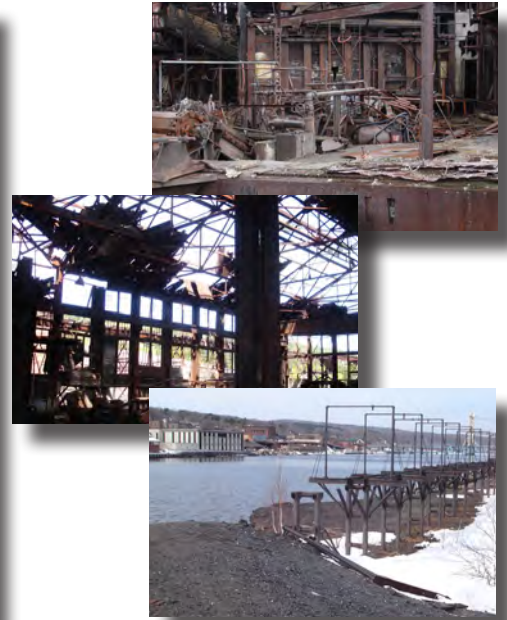
Abandoned materials, vacant buildings and infrastructure remnants.
