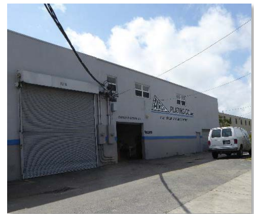
Figure 3. The front of the Airco Plating facility.
