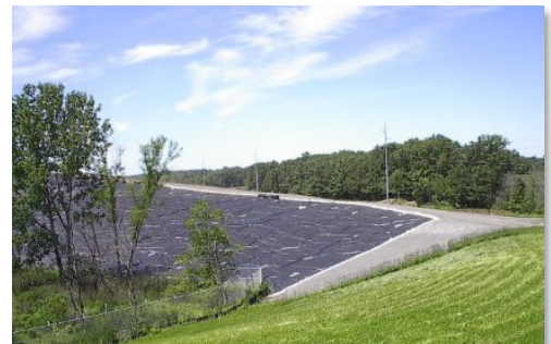
Figure 6. Construction of the cap over Shaffer Landfill.
