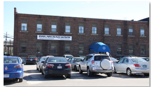
Figure 9. Pan Am Railways facility.
