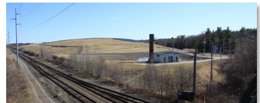
Figure 11. Shaffer Landfill, adjacent to the railroad.
