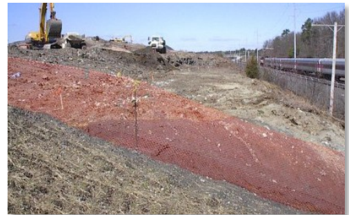
Figure 5. Slope grading on Shaffer Landfill.
