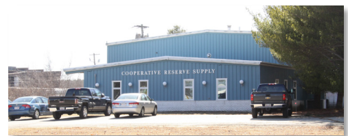
Figure 10. Cooperative Reserve Supply facility.
