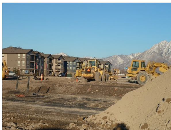
Figure 7. Site preparation for new development in 2011.
