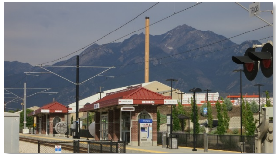
Figure 14. Bingham Junction's light rail station.
