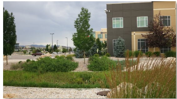
Figure 9. FLSmidth's facilities at the View 72 Corporate Center.
