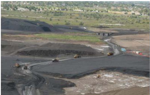
Figure 5. Cleanup activities at the Midvale Slag site.
