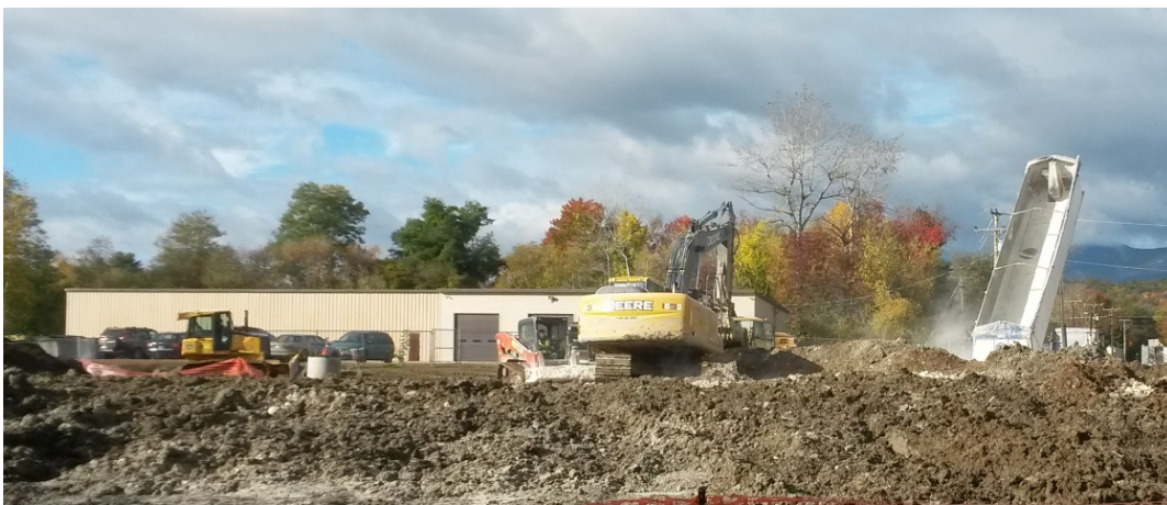
Figure 2. Soil cleanup underway, 2015.
