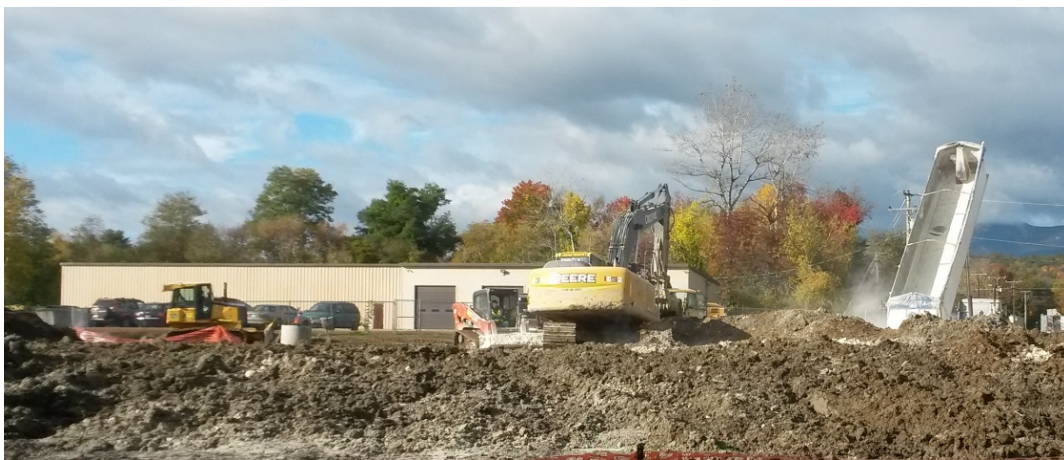
Figure 2. Soil cleanup underway, 2015.
