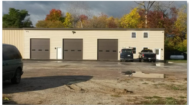
Figure 5. The former KMC building, now home to Hurteau Towing and Jon Hurteau Heating Services.
