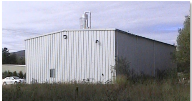
Figure 6. The former groundwater treatment building.
