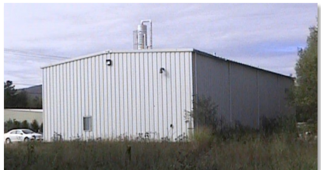
Figure 6. The former groundwater treatment building.
