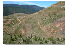
Erosion control – Bunker Hill Mining and Metallurgical Complex, Idaho
