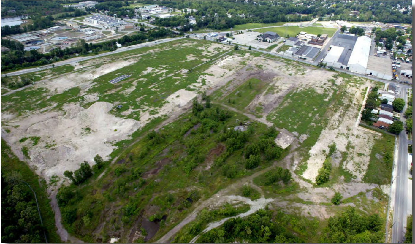
Future location of the site's solar array, 2003. (Source: Kokomo Tribune)
