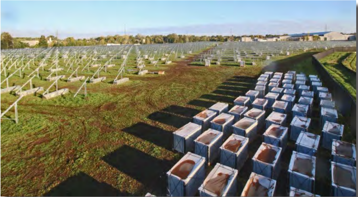
Preparations underway for solar panel installation, 2016. (Source: Inovateus Solar)
