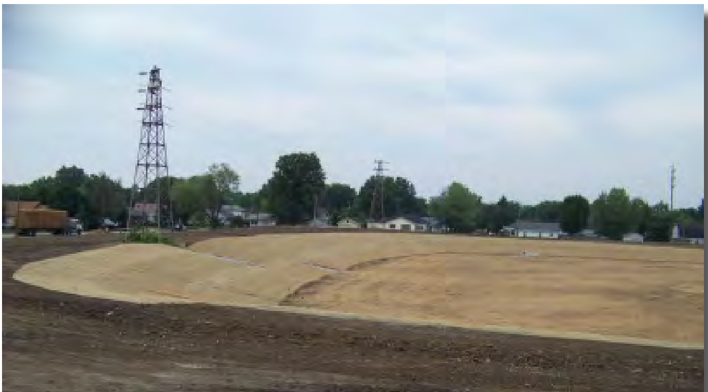
Stormwater retention pond on site. (Source: IDEM)
