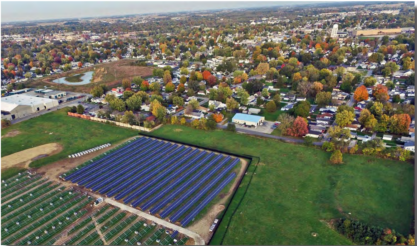
View of the solar array and surrounding areas. (Source: Inovateus Solar/Mike Robinson)
