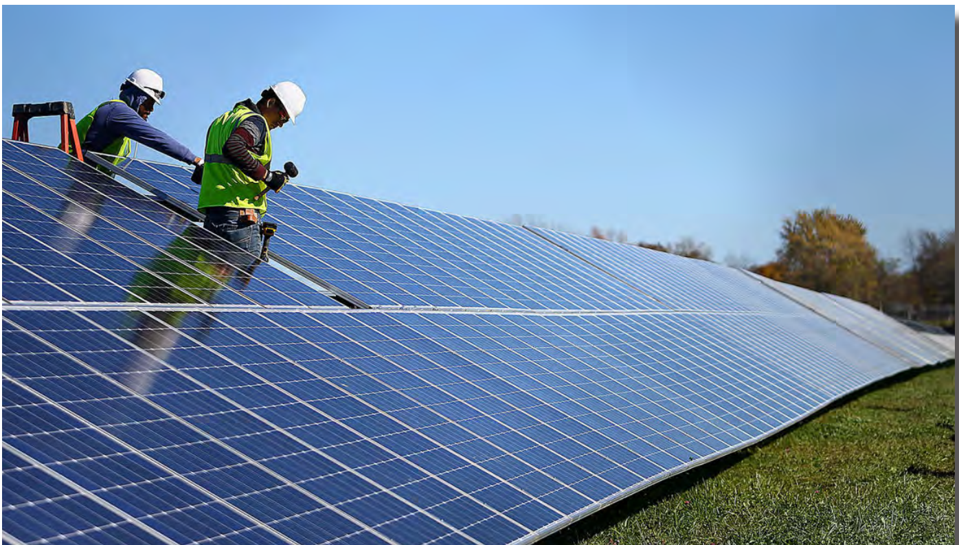
Workers installing a solar array, 2016. (Source: Kokomo Tribune photo)
