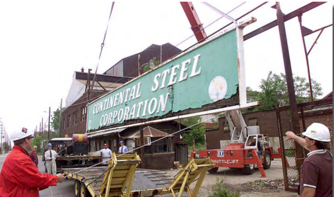
Company sign taken down in 1999, marking the beginning of building demolition efforts. (Source: Kokomo Tribune)
