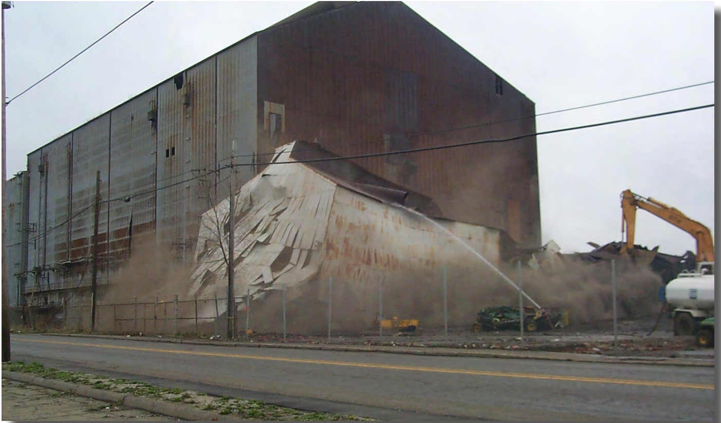
Furnace building demolition. (Source: IDEM)
