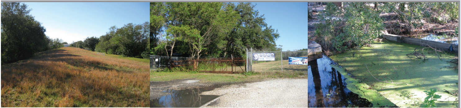
Images from left to right: View of the site's capped landfill, the entrance gate at North 58th Street, and a weir on the eastern edge of the eastern marsh.
