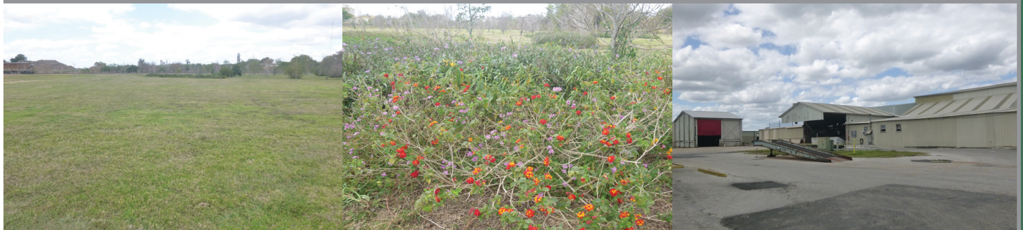
Images from left to right: Clay-capped area, pollinator garden and the Sylvite Southeast fertilizer-blending facility on site.
