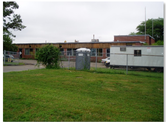
Figure 2. The former W.R. Grace building.
