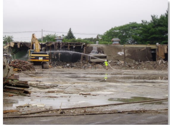
Figure 5. Demolition of the former W.R. Grace building in 2006.
