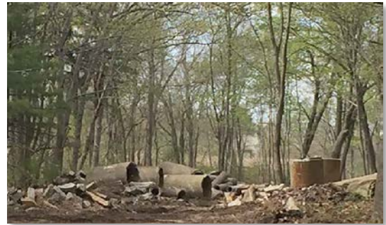
Figure 12. The City of Woburn property before cleanup and construction of the trail.
