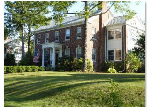
Figure 20. Renovated housing on site.
