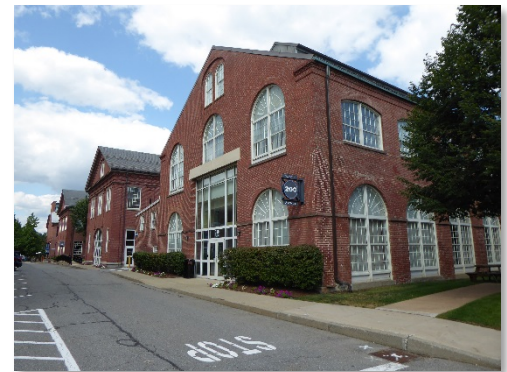
Figure 3. The former West Timber Storehouse was built in 1851. It is the oldest structure in the Arsenal on the Charles complex and currently occupied by office space, Bright Horizons and athenahealth.
