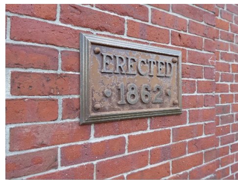
Figure 2. Built in 1862, Building 43 is one of the oldest buildings on site. Originally, it was part of the Seacoast Gun Carriage Complex.
