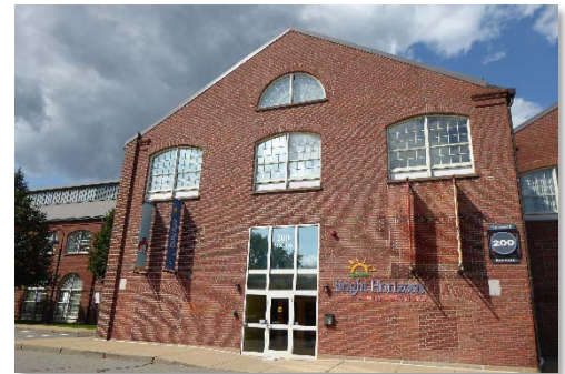
Figure 9. Bright Horizons is located at 200 Talcott Avenue, one of the oldest standing industrial buildings in the Arsenal.
