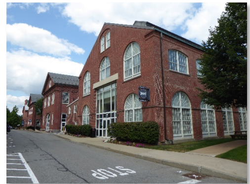
Figure 3. The former West Timber Storehouse was built in 1851. It is the oldest structure in the Arsenal on the Charles complex and currently occupied by office space, Bright Horizons and athenahealth.
