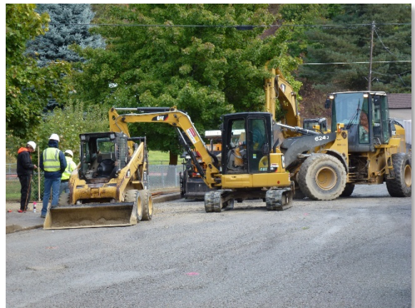
Figure 9. Utility and road infrastructure project underway in September 2017.
