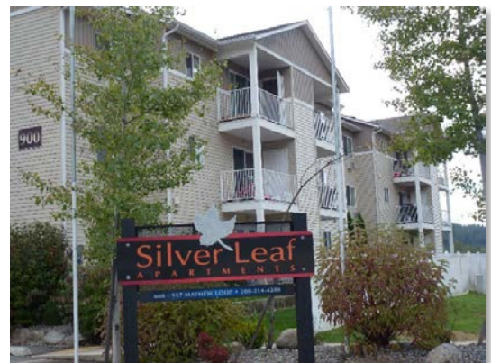
Figure 19. Silver Leaf Apartments at Smelterville Flats.
