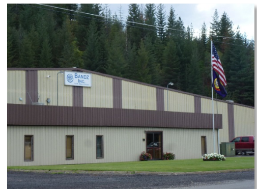
Figure 23. Examples of industrial and commercial use at the site.
