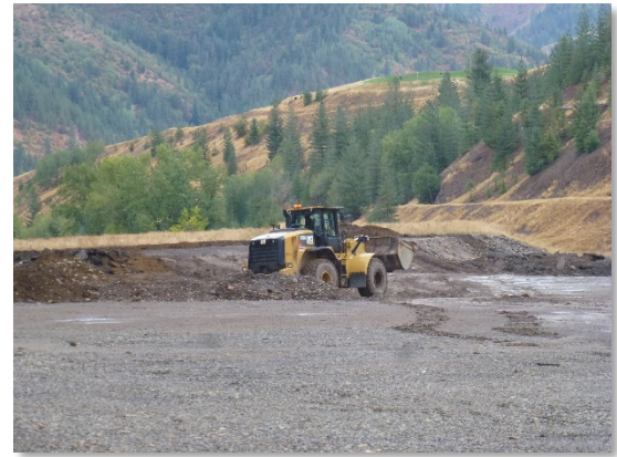
Figure 10. Improvements underway at Government Gulch.
