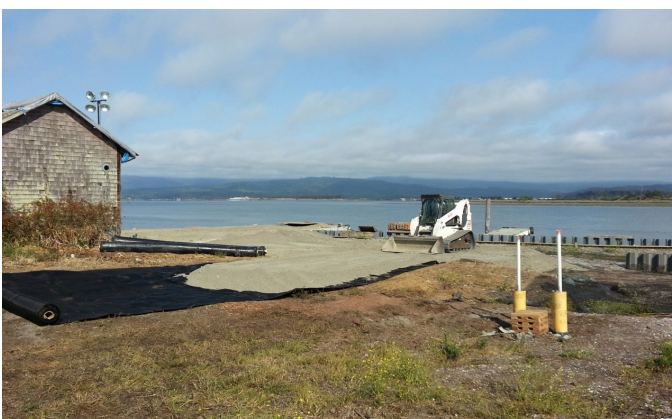
EPA strike team installing cap and placing clean fill at the site.
