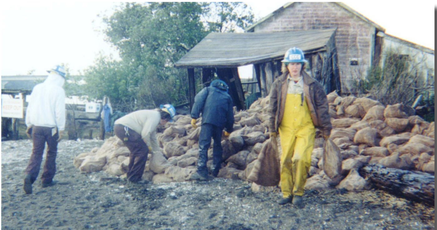
Workers using oyster shells for erosion control.
