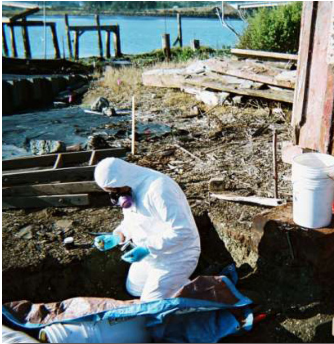
Each barrel of contaminated soil was filled and weighed by hand.
