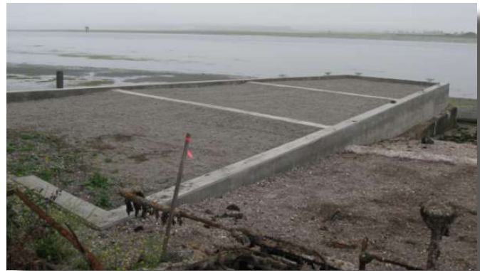
A total of 220 linear feet of sheet pile at the site prevents erosion, protecting the shell midden and other cultural and environmental resources.
