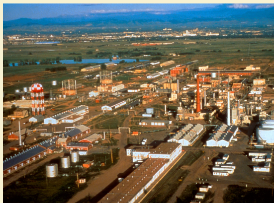
Top: Women working at the South Plants, 1952. Above: South Plants prior to demolition. Images used with permission of the Army.
