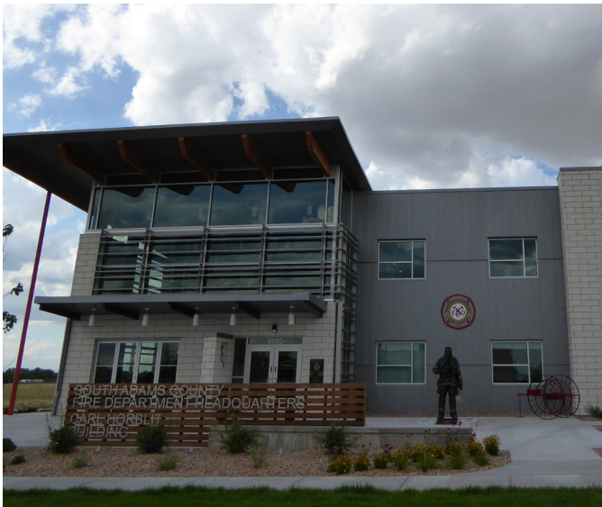
The new South Adams County Fire District headquarters is located on the Western Tier Parcel.
