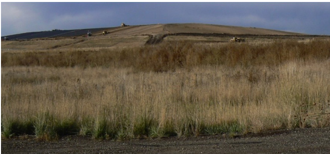
Above left: The landfill cover was carefully graded so the area would blend in with the surrounding landscape.
