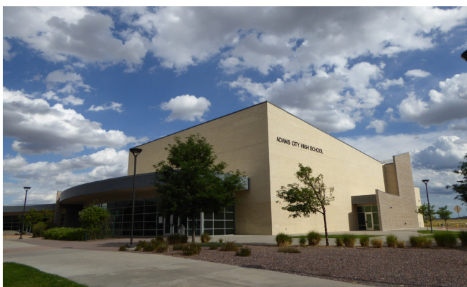
Community amenities built on the Western Tier Parcel include the Commerce City Civic Center and Adams City High School.
