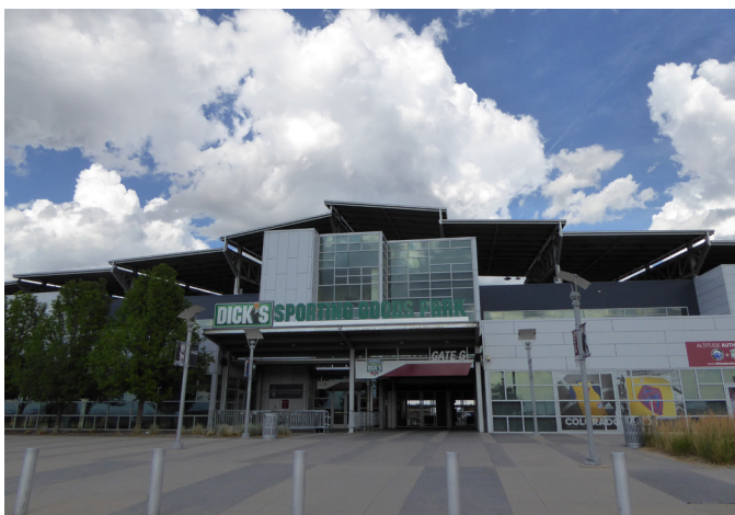
Dick's Sporting Goods Arena is part of a massive soccer complex at the site.
