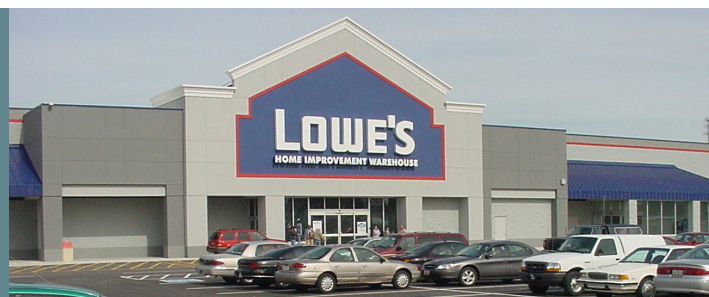
Figure 15: Prestolite Battery Division site (Indiana)
