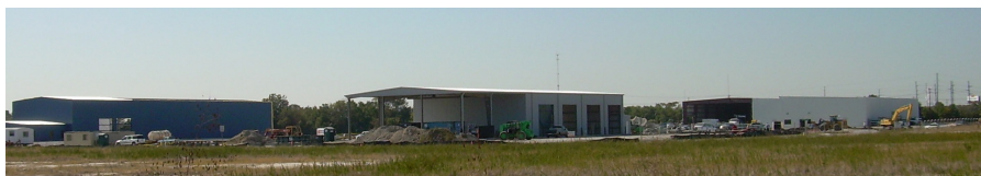
Figure 7: Macalloy Corporation Superfund site (South Carolina)
