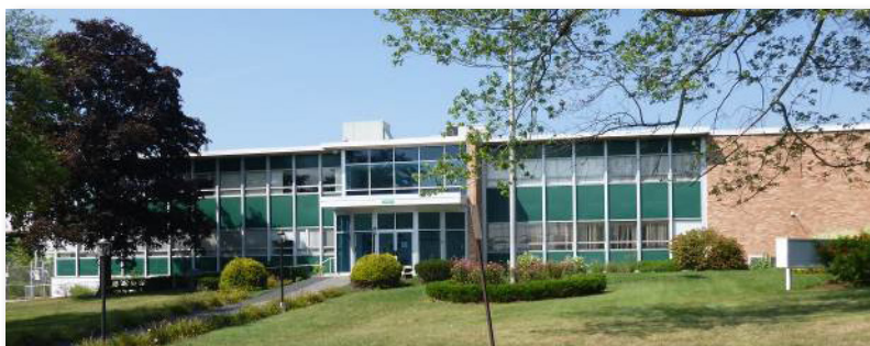
Figure 11: The former Peterson/Puritan facility remains in use today. The parcel contains a groundwater pump-and-treat and soil vapor extraction operation.
