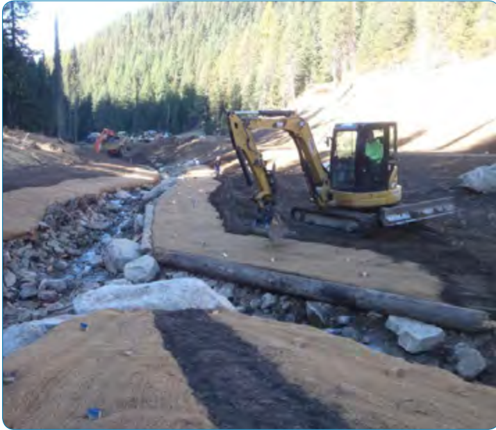
Crews constructing a new stable channel in the cleaned up area.
