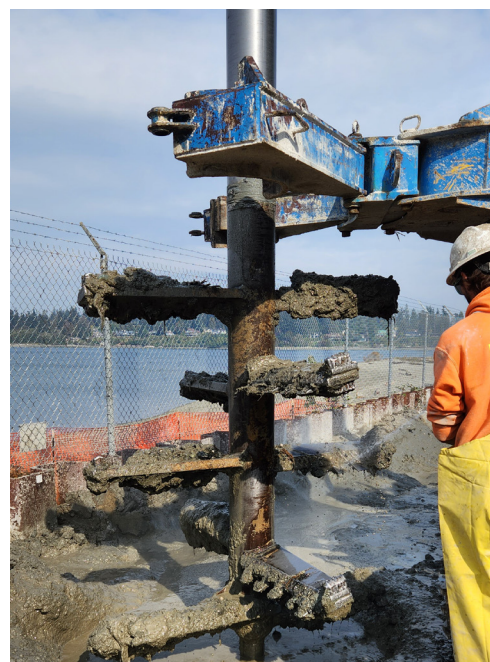
Augers mixing cement into soil during ISS (Jacobs Engineering Photo)
