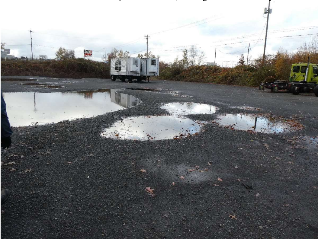
Former impoundment area, with truck storage and ponding
