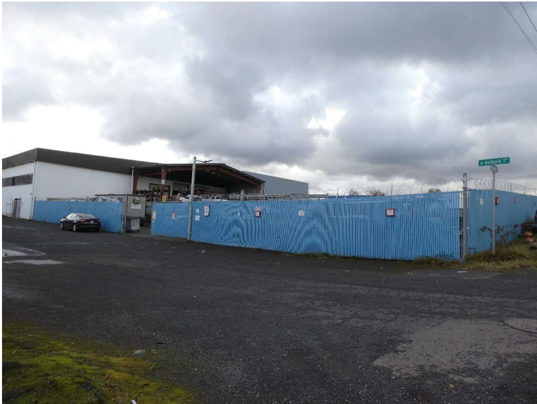
Fenced portion of former administrative building area
