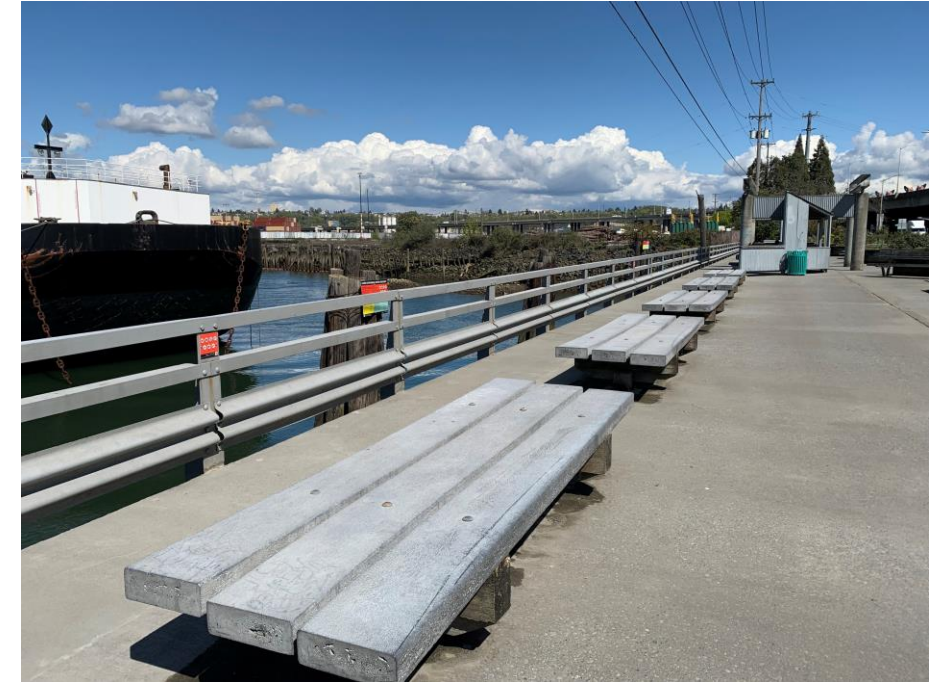
View of Spokane Street Bridge (over the East Waterway)
