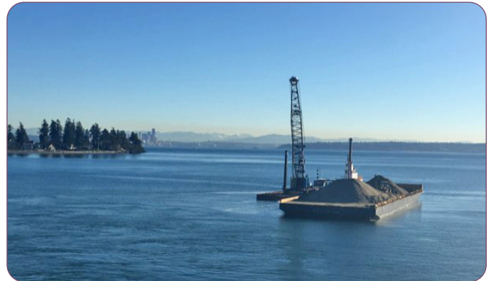
In 2017, EPA repaired the subtidal cap.
