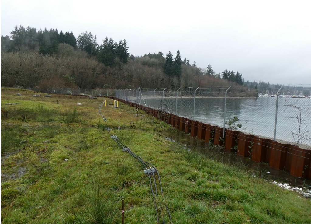
Interior sheet pile wall with West Beach visible in background
