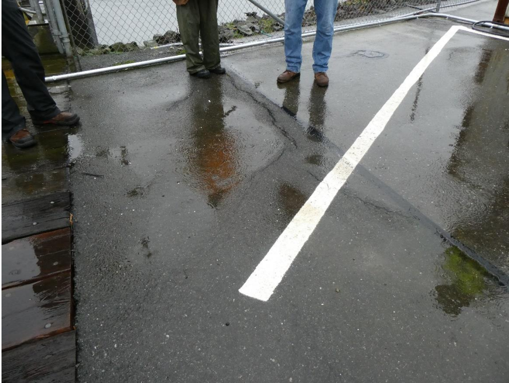
Asphalt crack repair
