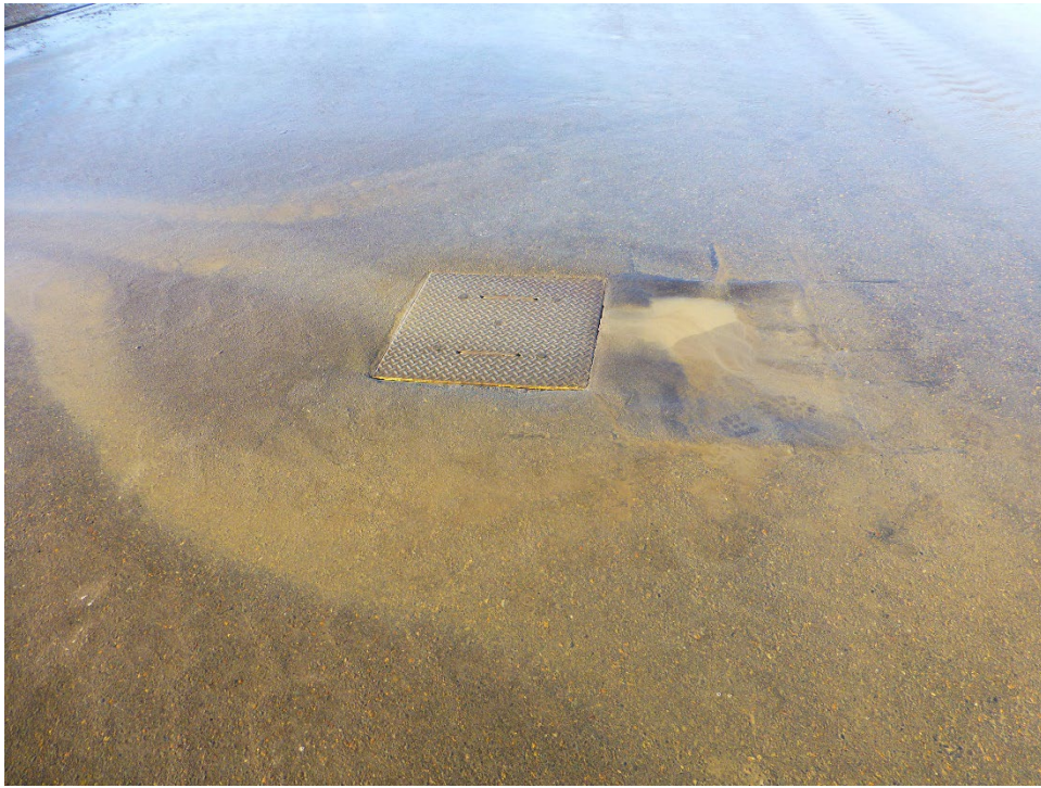
Groundwater extraction well PW-4
