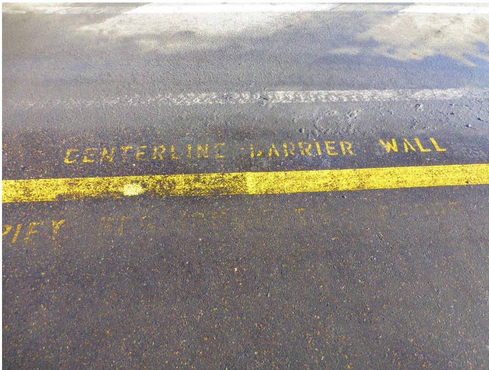
Painted yellow line marking subsurface barrier wall
