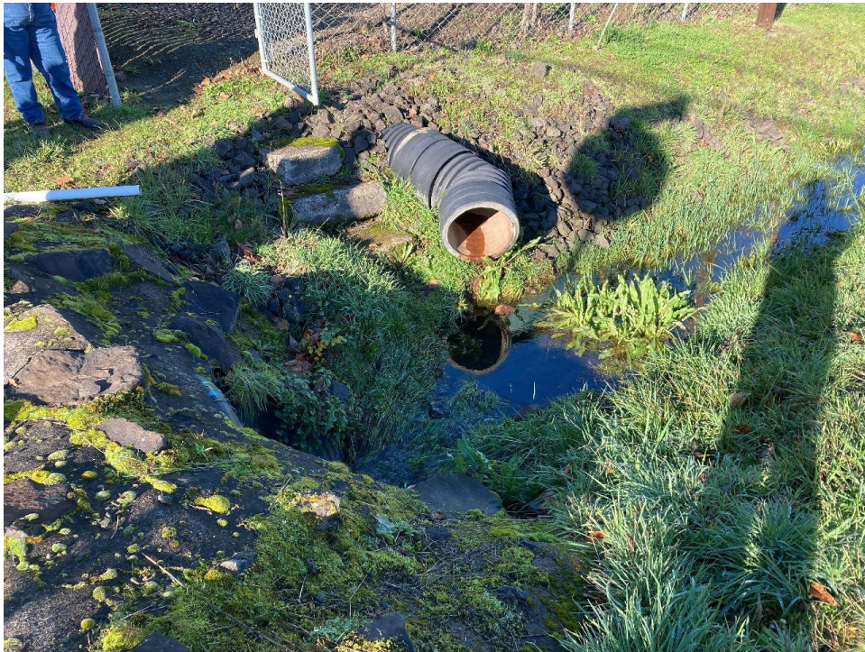
Outflow 003 discharging treated water
