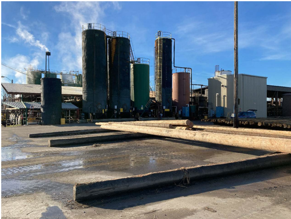
Structures for wood-treating operations
