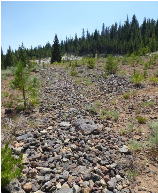
Stormwater diversion ditch on Lucky Lass stockpile
